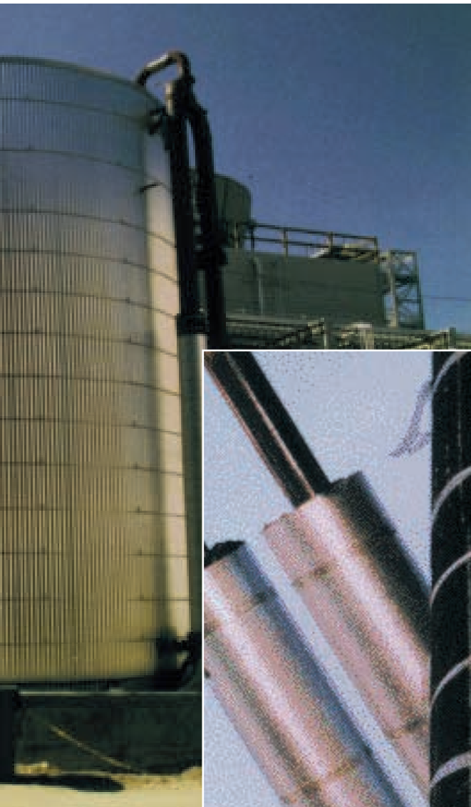
Pipe sizes range from 1/2-inch- to 36-inches in diameter, with most being in the 4- to 6-inch range. FOAMGLAS® Super K™ insulation was prefabricated in 2-foot, half-round sections and field applied, in thickness ranging from 2- to 3-inches, secured with stainless steel strapping and covered with corrugated aluminum jacketing.
