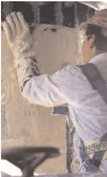
For cold processing equipment requiring a vapor barrier, a mastic was applied to FOAMGLAS® Super K™ insulation and the lines were covered with aluminum jacketing.
